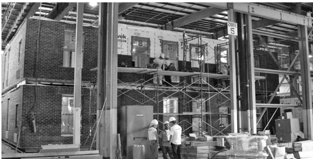
Fig. 1. Module production of a 3-story dormitory project
